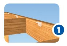
Step 1: Starting from the outside, attach the Invisi-Fast™ with no spacer between each joist. \*Install first board with proper overhang and secure using the top holes (Deck Board Holes) of the Invisi-Fast™ fastener.
