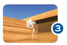
Step 3: Secure the deck board by using the corresponding upper hole. Slide your second board into place. Secure deck board by using the remaining upper hole.
